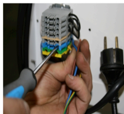
5 Connect power and remote humidostat wires.
