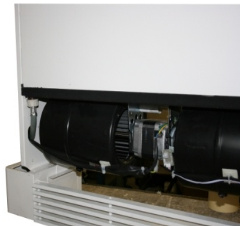
5 Connect power and remote humidostat wires.
